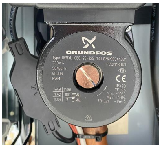
Grundfoss Pumpe UPMXL GEO 25-125 130 PWM
